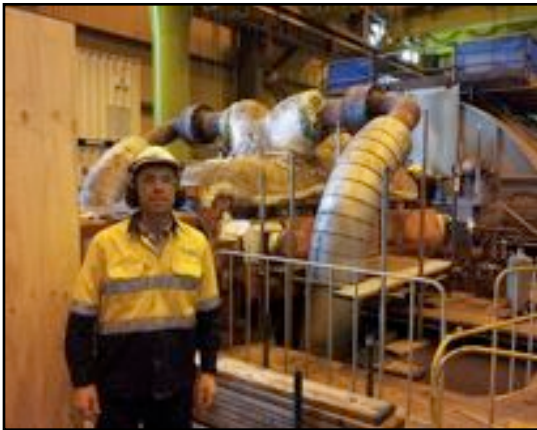
John by Unit 1 Turbine during disassembly
