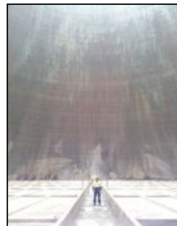
John inside one of the two Cooling Towers during the Loy Yang B outage
